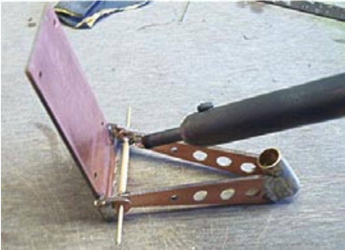
Solder the 3/32" brass pivot tube to the supports.
